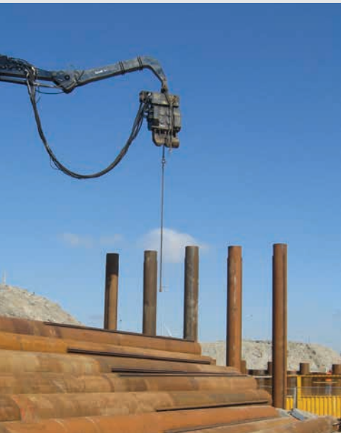
Combined Wall with pipes and Larssen U-section Connector L8
