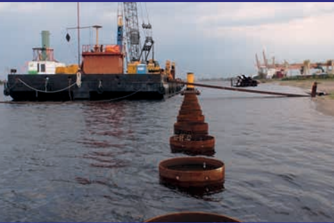
Combined wall with pipes and Z-Section with Connector LPB 100
